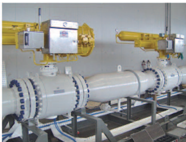
CB54 gas plant installation
